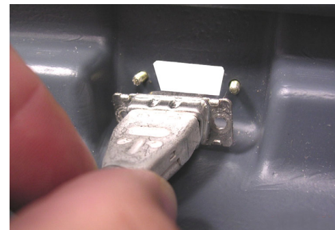
Installing New Pigtail
